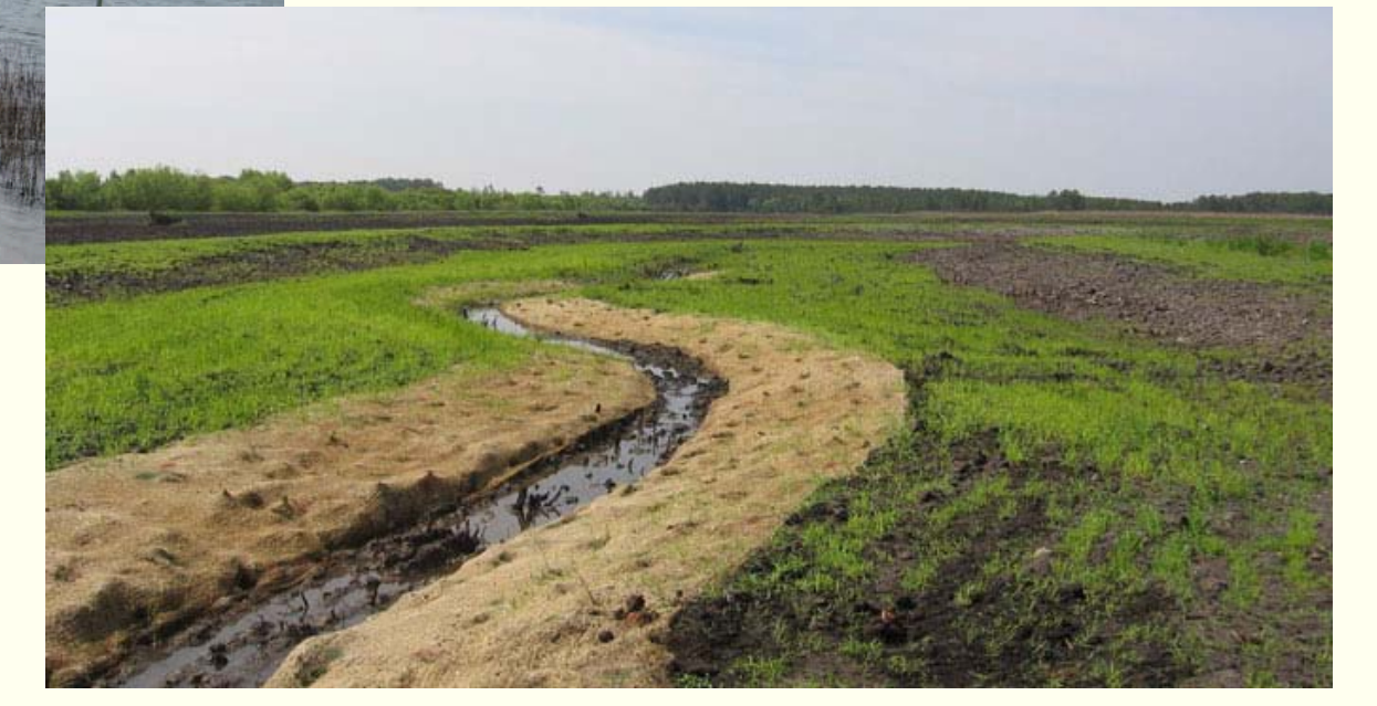
Figure 8. North River Farms restoration project (Source: North Carolina Coastal Federation website)
