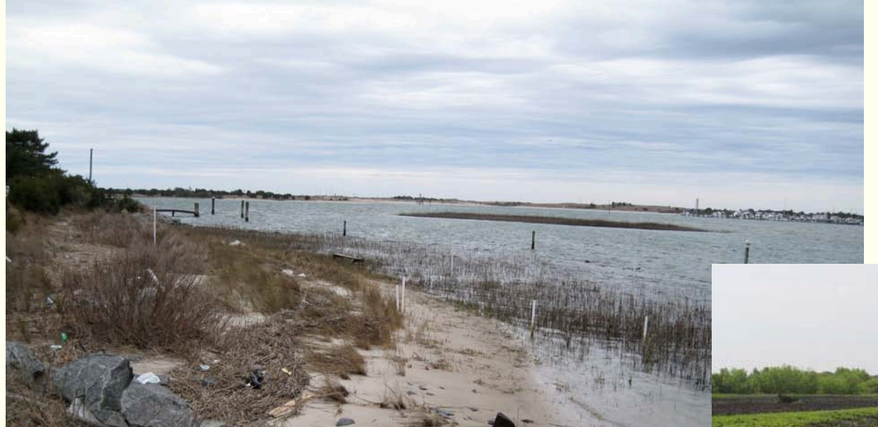
Figure 7. Example of living shoreline, Beaufort, N.C. (Photo Courtesy of Arleen O'Donnell, ERG)
