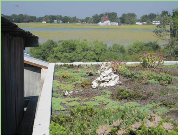
Green roof, Bowens Island
