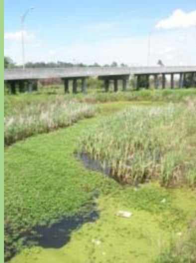
Constructed wetland, SCDOT Rivers Avenue
